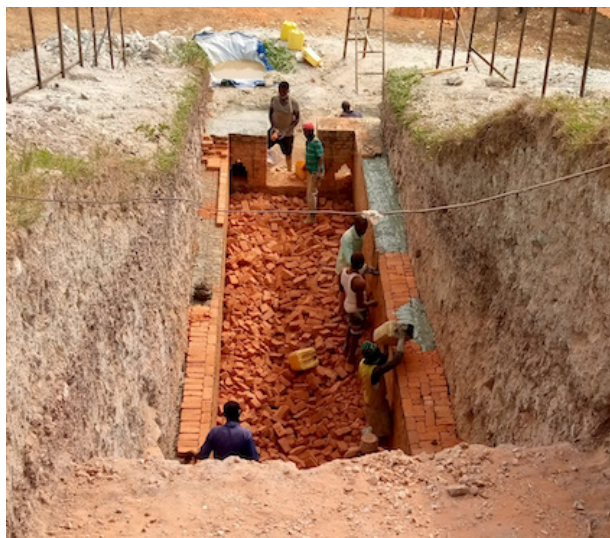
Trench kiln under construction. Recycled fired bricks serve as insulating wall and floor surfaces.
